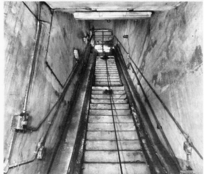
The main access stairs into the bunker. Photo Nick Catford SOURCE: Bucks Free Press , 15 March 2012
